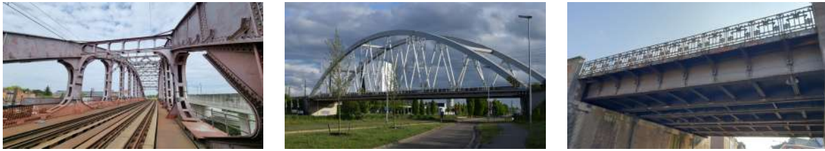
Figure 1: Left: The Vierendeel arch bridge (Mechelen, Belgium). Center: The KW51 tied-arch bridge (Leuven, Belgium). Right: The Nieuwebrugstraat riveted beam bridge (Ronse, Belgium).
